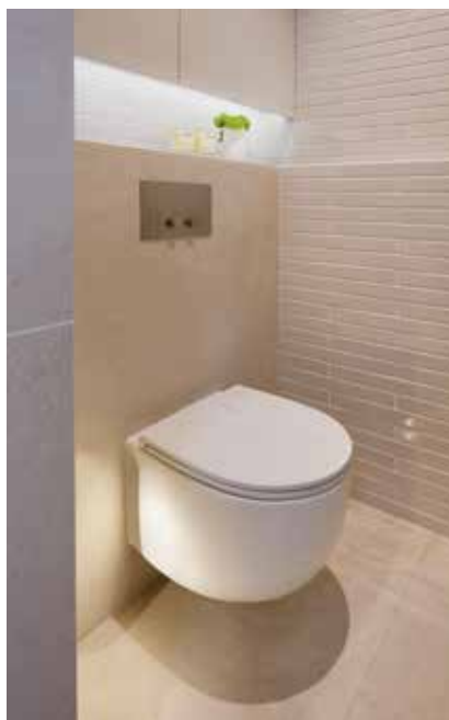
The WC , from West One Bathrooms, was kept close to the soil stack, but positioned around the wall to give added privacy. Flush plate, Fantini.
